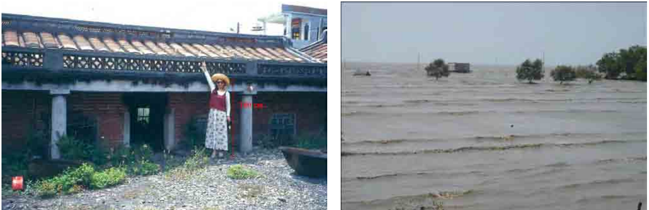
Figure 2.2.2. (a) A house in an area where land subsidence is severe due to overpumping of groundwater (picture by C.T. A. Chen). (b) Land with telephone poles has become submerged due to subsidence (picture by Ajira Tiangtrong).
